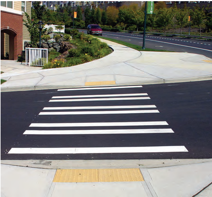
Accessible street crossing at an unsignalized intersection
