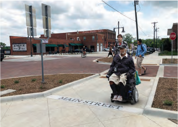
Streetscape with accessible curb ramps and street crossing
