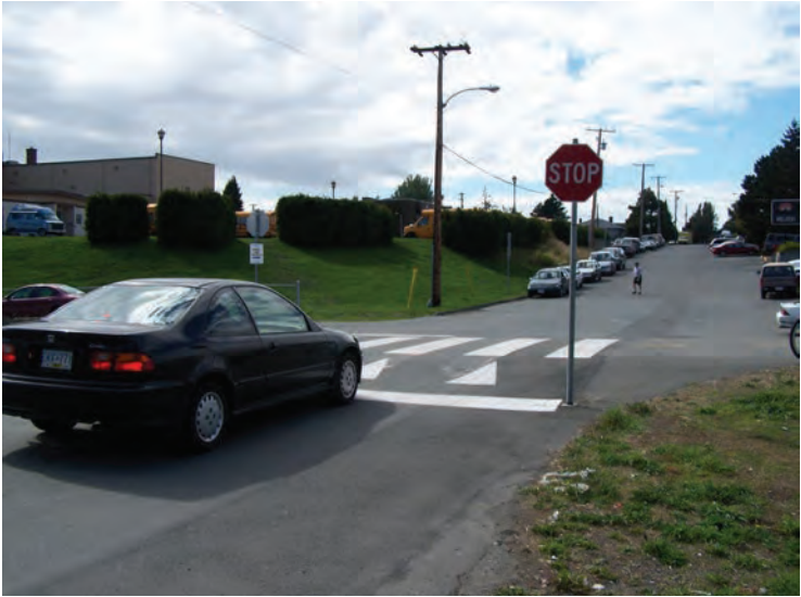
Raised crosswalk at an unsignalized intersection.
