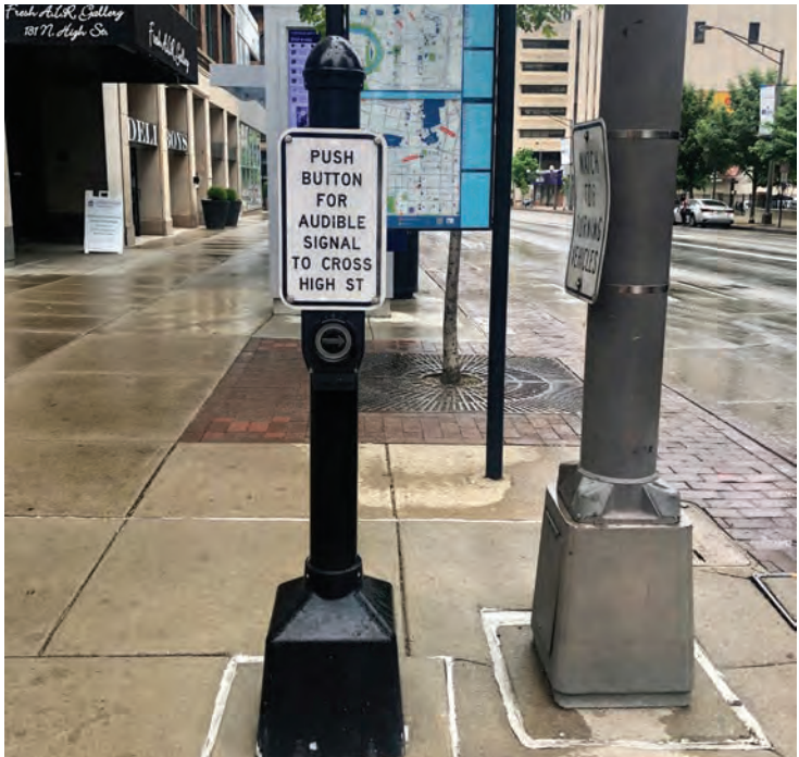
Accessible pedestrian signal button and signage
