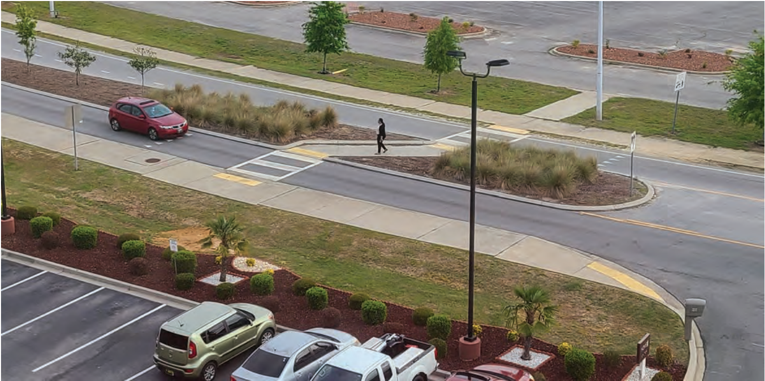
Raised crosswalk at an unsignalized intersection
